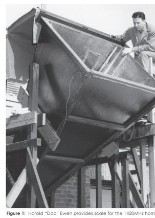
**Figure 1:** Harold "Doc" Ewen provides scale for the 1420MHz horn antenna, made from copper-clad plywood, on the parapet outside Lyman 4th floor. The canvas cover was added after the horn funneled a rainstorm into the lab (which Ewen remarked was his first "signal from space").
