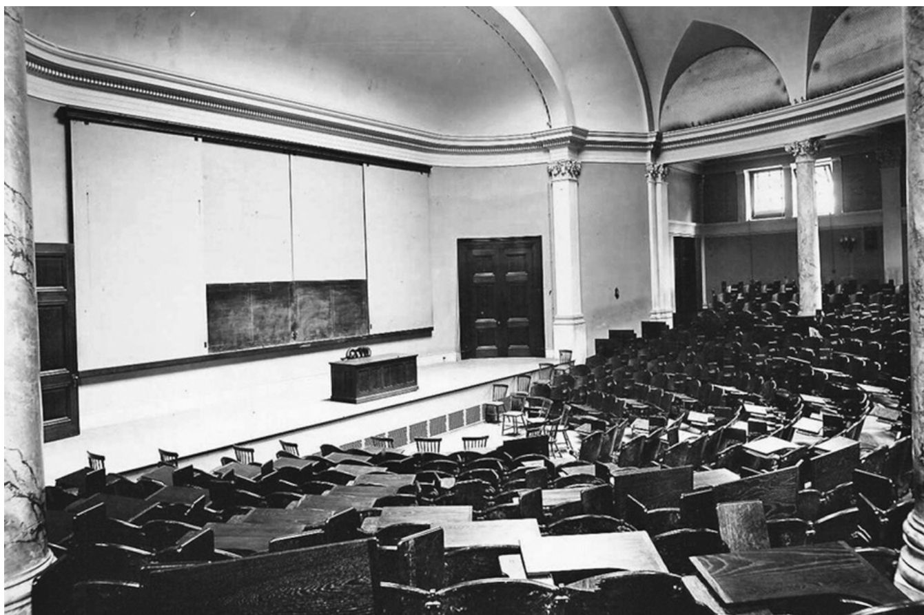
Fig. 2: The new Fogg lecture hall, circa 1895, where lectures were unintelligible. Note the hard surfaces, such as plaster walls and ceiling, and hard-surface student desks and seats; evidently it occurred to no one to equip the latter with cushions.
